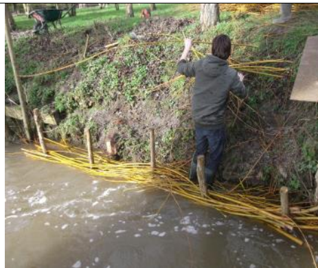
Weaving willow branches in acordance with the current flow
